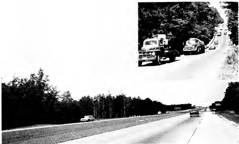
Dualization of U. S. 301 in Southern Maryland is progressing. This is a completed section in Charles County. The inset shows a section of the old road where one slow-moving vehicle could hold up a line of cars.
